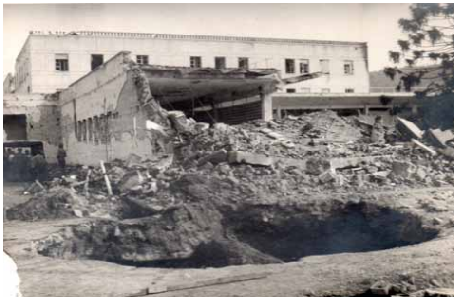
A view of the 45th General Hospital's area when it arrived in Naples on 19 December 1943. A bomb crater is in the foreground. This building was repaired enough to house the most serious patient cases.
