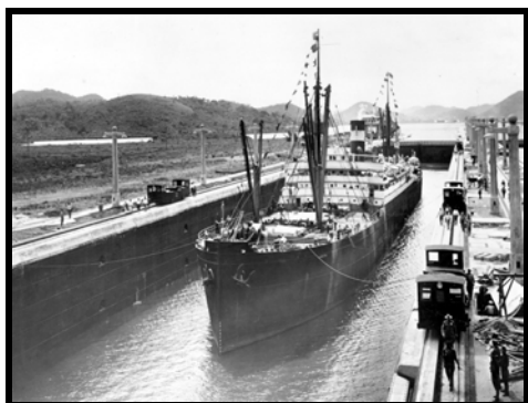
Naval Vessel Transiting Panama Canal, 1941
