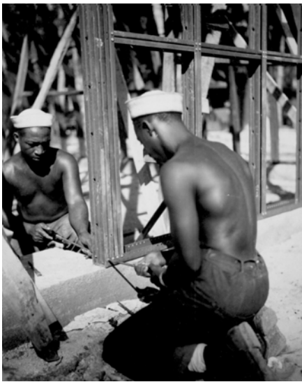
Construction of a prefabricated steel storage warehouse by members of the 34th Construction Battalion in South Pacific during WWII. Photo courtesy of National Archives.
