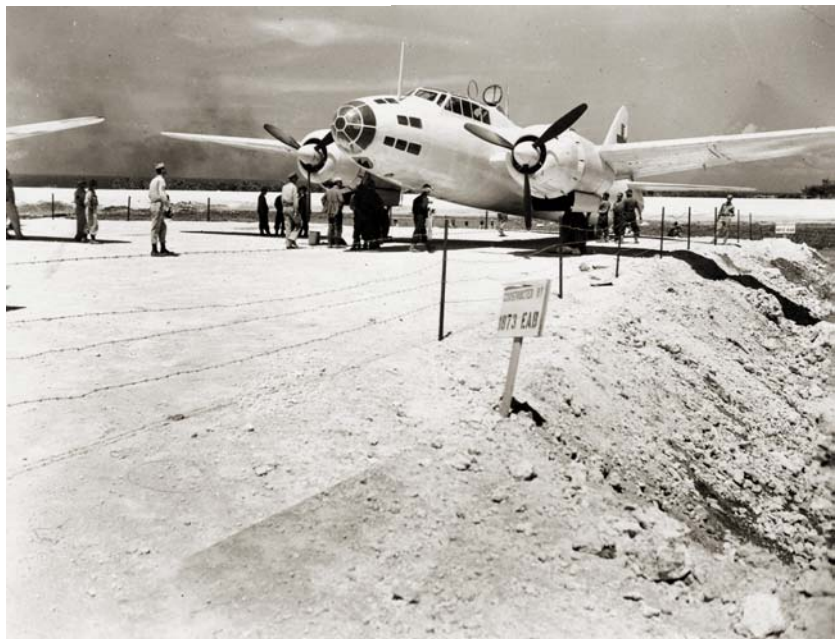
A runway on Ie Shima constructed by the 1873rd EAB. It was also where the Japanese military and civilian envoys landed on 19 August 1945 to change planes. The Japanese party was enroute to General MacArthur's headquarters in Manila to receive instructions concerning surrender and occupation arrangements.
