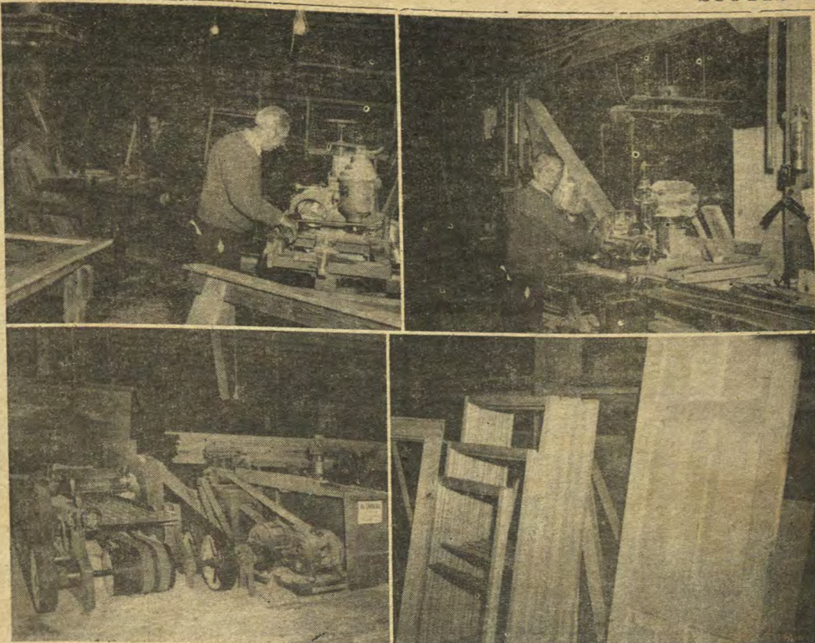
Haden Anderson operates shaper as J. H. Duncan works with Tenon machine at W. F. Paulett and Co. in the upper left photo. Mr. Duncan is shown operating combine cutoff saw in upper right picture. Lower left photo shows planer and cutoff saw while lower right shows finished product of mill. (AEP Co. Photos)
